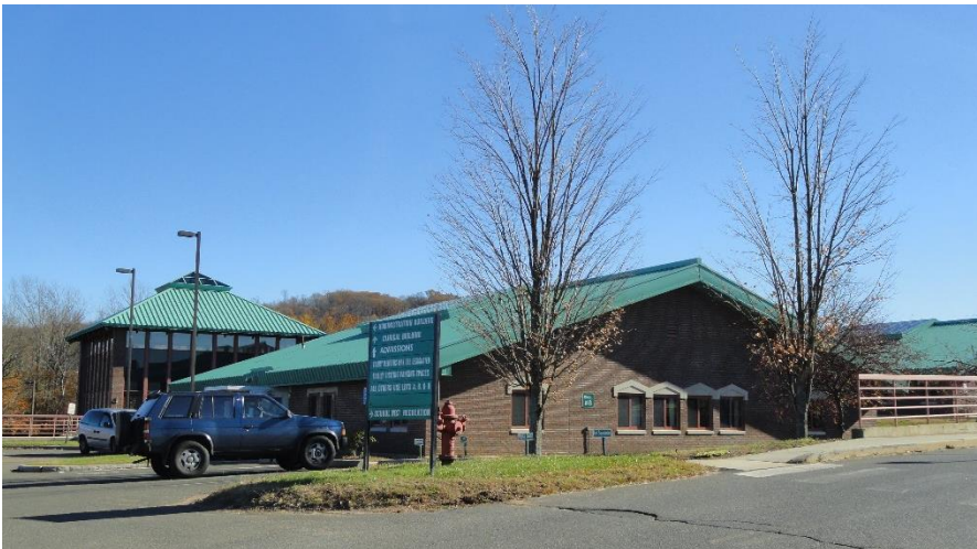
Albert J. Solnit Children's Center – South Campus
