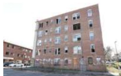
Courtland Arms building
