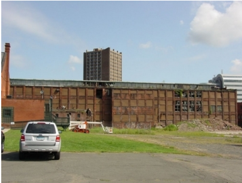
Former Capewell Horsenails Factory
